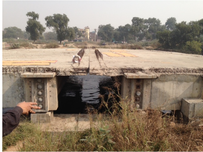
Fig. 1. View of the well cap and deck of bridge under construction
